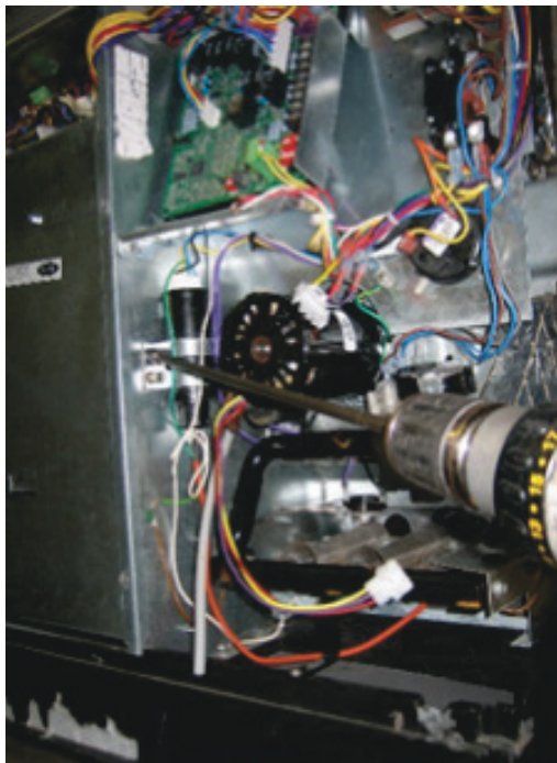
Fig. 31 – Removing Mounting Screw from Gas Manifold A210076
