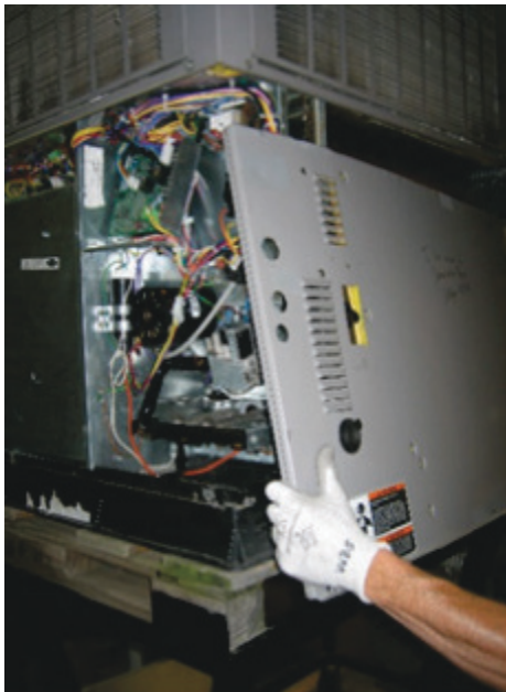
Fig. 36 – Replacing Right Side Panel
